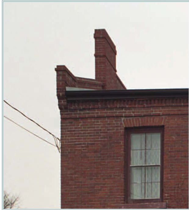
This house is a fine example of the urban townhouse style characterized by blind parapet walls.
