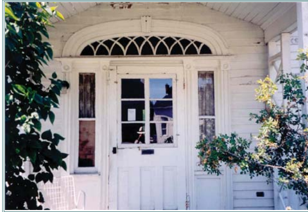
On the main facade, under an open portico, sits the main entrance in a detailed surround. The trim is fluted and decorated with medallioned corner blocks. Above the door is an arched, light transom with curved muntins. A moulded keystone crowns the fine architrave above.
