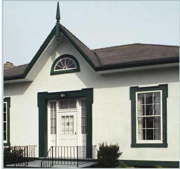
The door case and windows both have an 'eared' corner moulded trim, which are details typical of the Classical Revival period circa 1830-1860.
