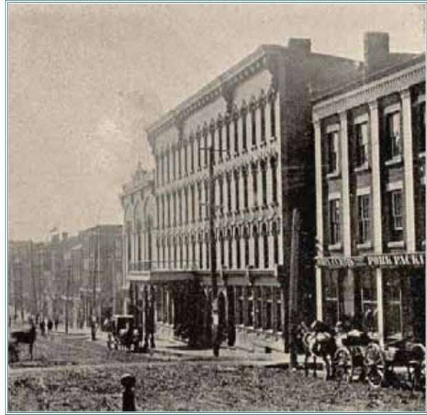
The Porter Block was built before the neighbouring St. Lawrence Hall. As seen in archival photos, the building was a handsome block with contrasting pilasters and projecting brick caps with ornamental brick cornice to eaves. The shop fronts were typical of commercial buildings of this period.
