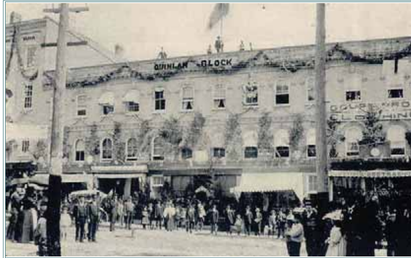
The Quinlan Block decorated for an event at the turn of the century. The building represents the third phase of Walton Street building with pilasters absent but complex decorative brickwork of band courses, window labels and cornice topped by panelled brick parapet.
