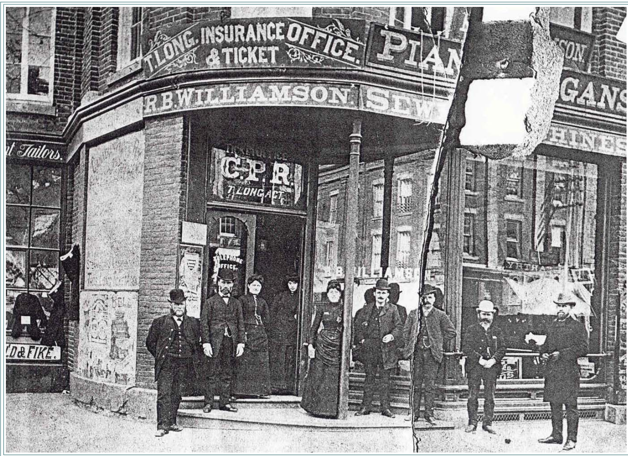
The entrance to 35 Walton Street was on the rounded corner of the building. Photographs from the Clayton Collection place Merrifield and Fike, merchant tailors, in the shop facing Queen Street during the tenancy of Tom Long Insurance and R.B. Williamson.
