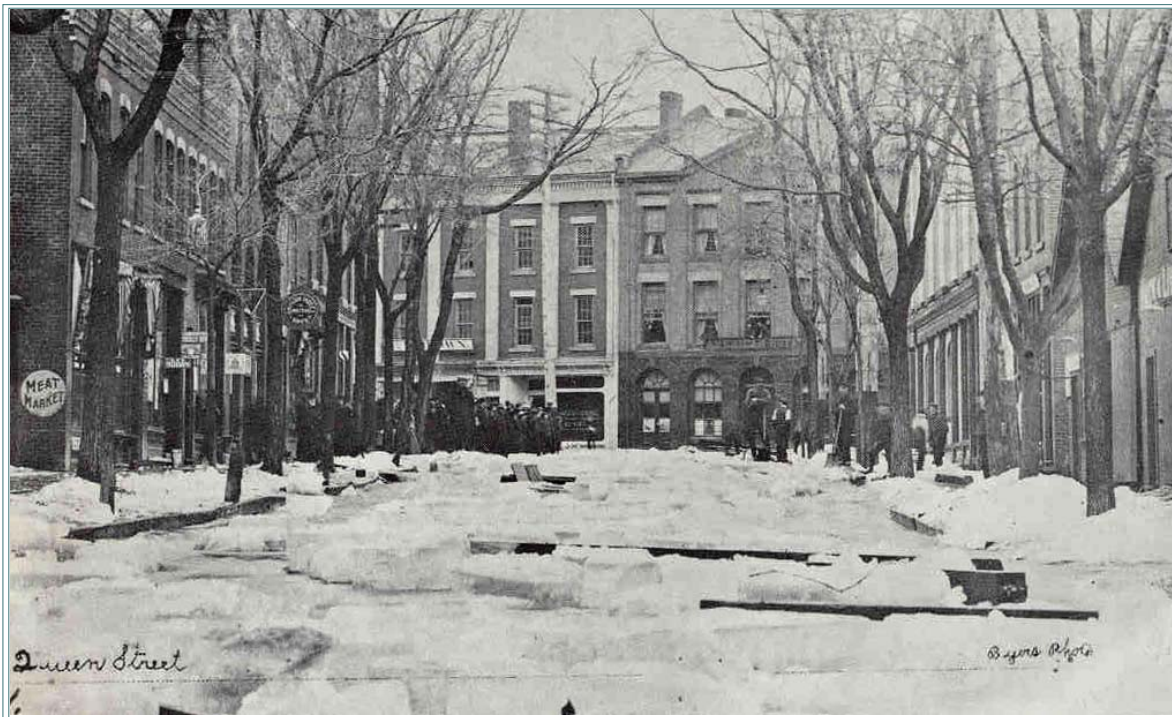
A view of the North American Hotel as a focal point from Queen Street with its original arcaded lower storey.
