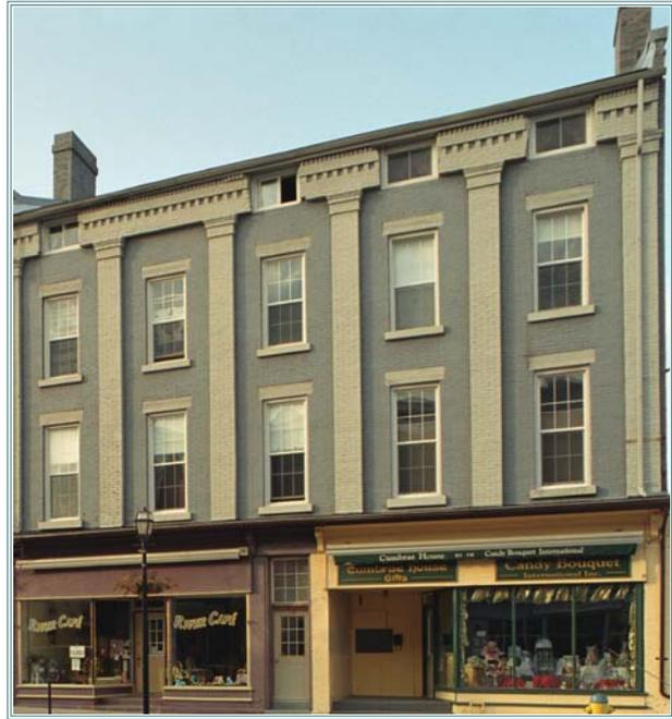
*The mid-19th century block with ornamental brickwork to cornice and frieze has been altered by later windows punched through the wall to light the attic storey in the eastern three quarters of the block.*
