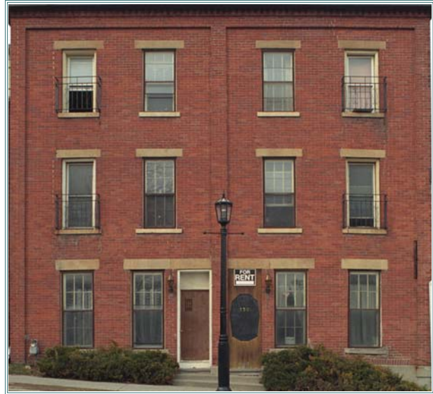
Perks Terrace is a three storey, four bay commercial type block of the transitional type with plain pilasters and frieze outlining the two units.
