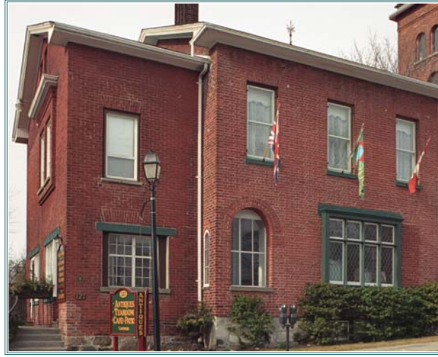
Originally the main facade had three bays on the first and second storeys. The extension to the east housed a medical office. The roof was parapet gabled, similar to numerous other Port Hope dwellings of the townhouse type.
