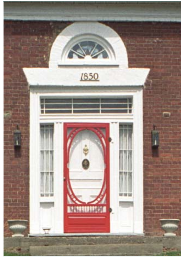
Rectangular multi-paned sidelights and a transom of the same style and dimension flank the fine Palladian proportioned front entrance. A unique fanlight window that provides light to the upper storey appears to rest on the door lintel.
