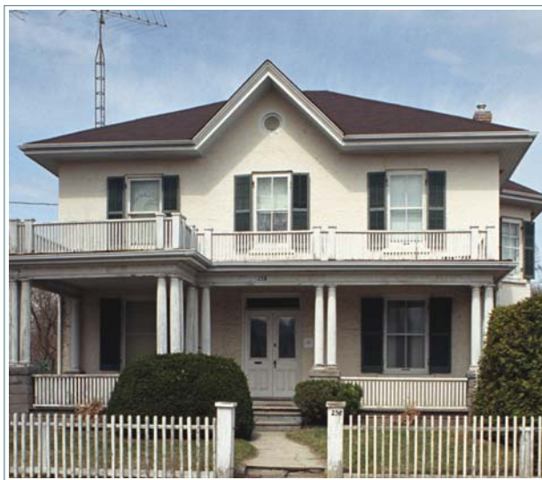
This is a three-bay house, with a centre-hall plan. The large windows are two-over-two and double-hung. They sit on either side of the central opening on both storeys.
