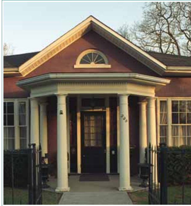
The front entrance is graced by a semi octagonal wood portico of generous dimensions.
