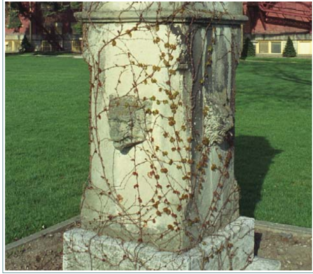
When functioning water pours from the mouth of each lion head in a stream originally into a trough below.
