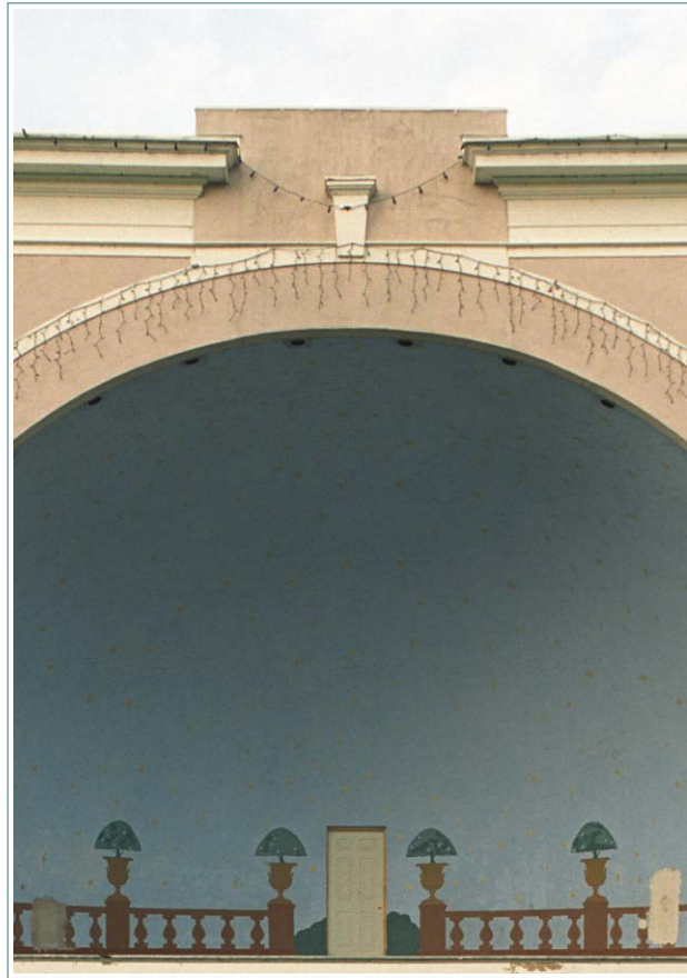
The Memorial Bandshell incorporates many classical features including the keystone and ornate heavy cornice.
