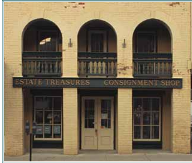
The existing recessed shop front was installed circa 1930 by the Strong family. Prior to that time, two equally spaced brick columns came down to grade from the arches above. See archival photo detail below.
