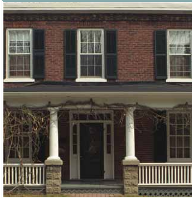
The balanced facade and transomed door suggest a Regency style, whereas the roof is flat and slopes gently to the rear which is more of a townhouse detail.
