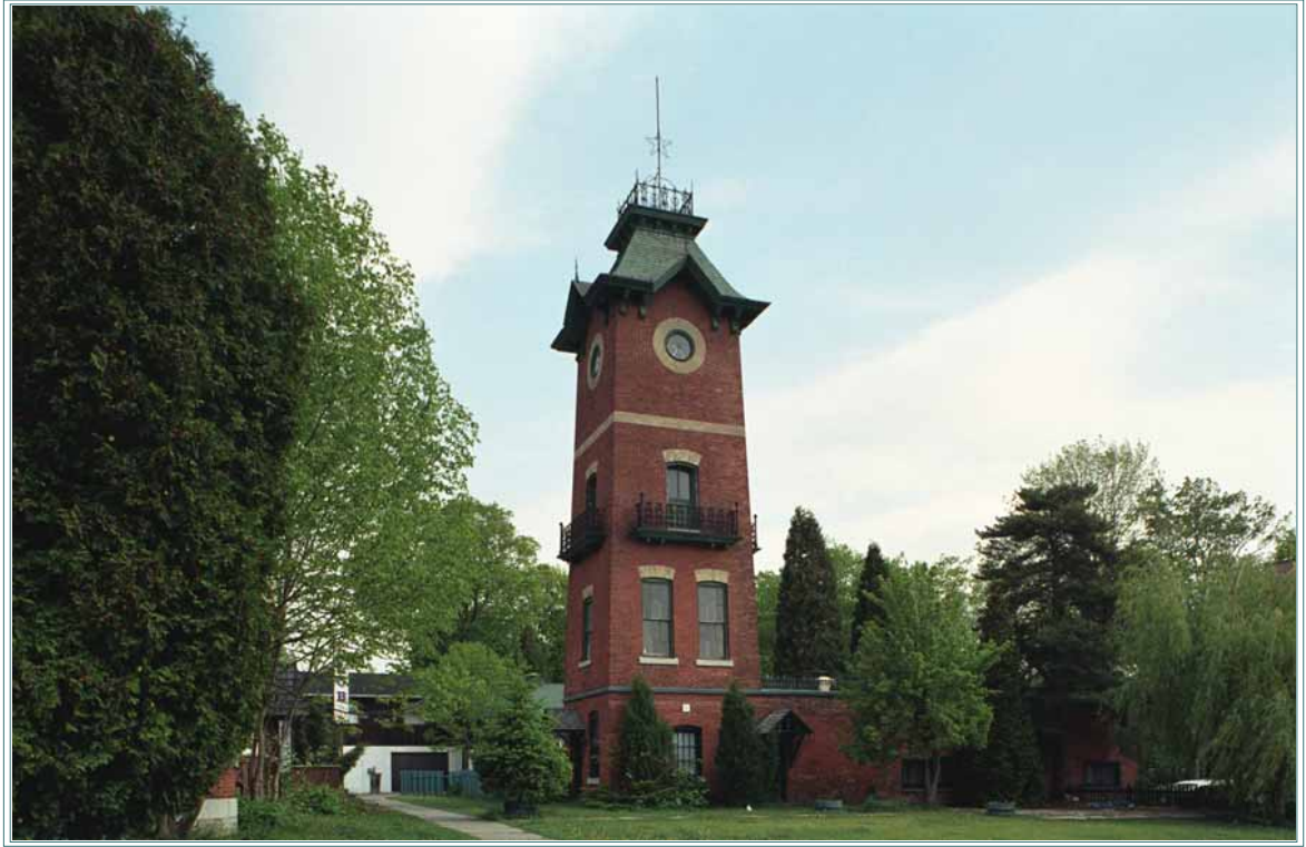
JOHN HELM JR. HOUSE (BELGRAVE) WATER TOWER circa 1877
