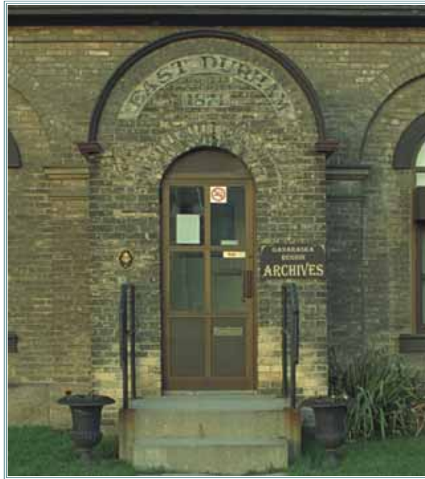
The barrel-vaulted entranceway is thought to be a later addition.
