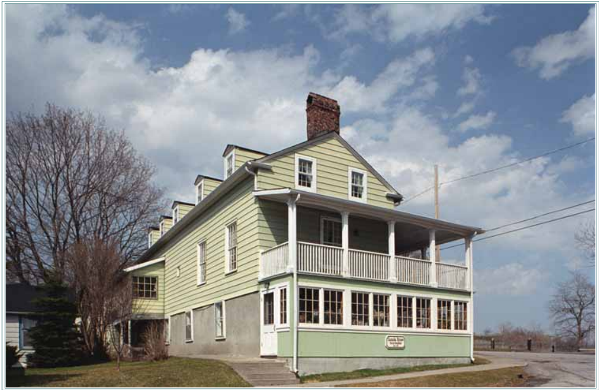
ELIAS SMITH HOUSE (CANADA HOUSE) circa 1800 (RESTORED)
