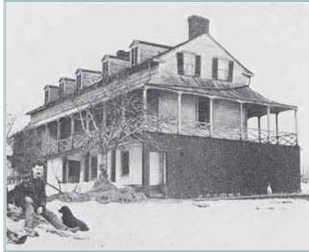
Evident in this archival photo, the verandah at one time extended around three sides of the building.
