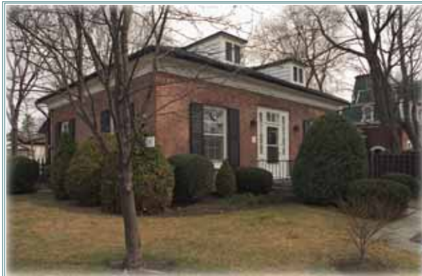
The brick house has one and one half storeys, a centre door, and two large first floor windows on either side of the front door, and a low hip roof with two front dormers.
