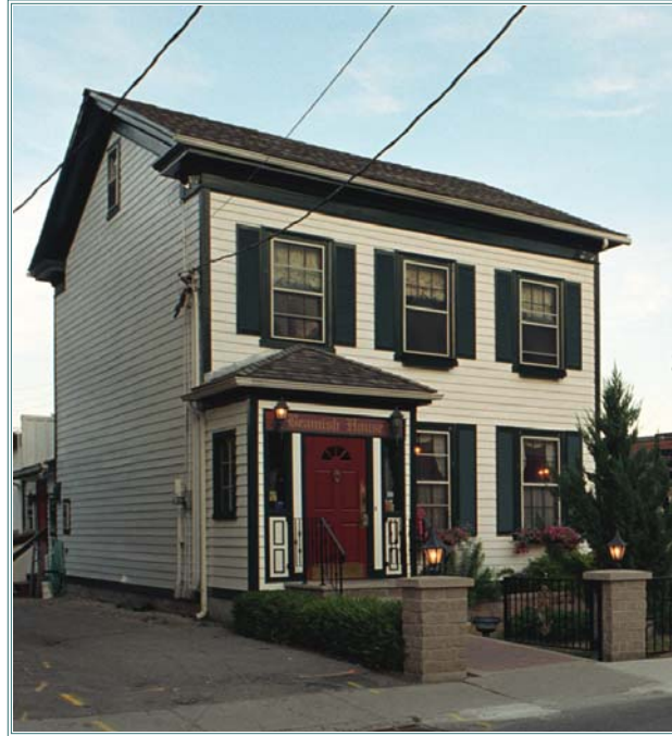
On the gable ends are wide returned eaves, a feature of the Classic Revival style.
