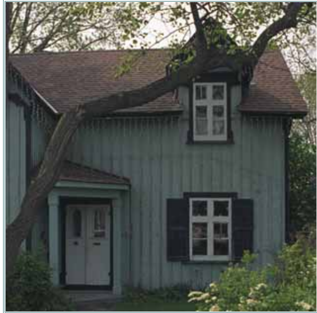
Early photographs reveal that a porch ran the length of the west half of the facade.
