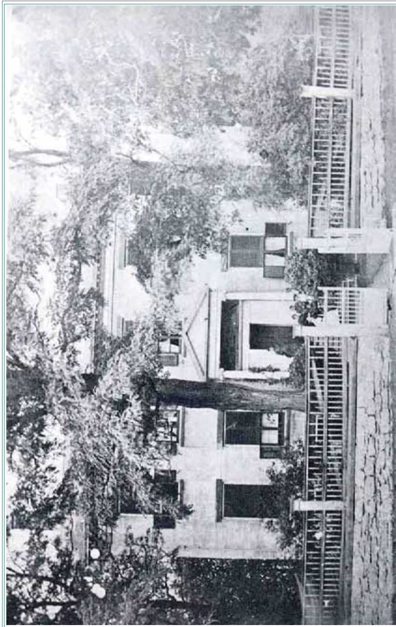
A view of the Bluestone enclosed behind a fence with sectional shutters both open and closed and with a seasonal entrance enclosure under the front porch.
