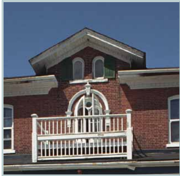
This central window is essentially a pair of narrow round-headed doors or French windows set into an opening with a centre lozenge, the whole device resulting in a Florentine window.
