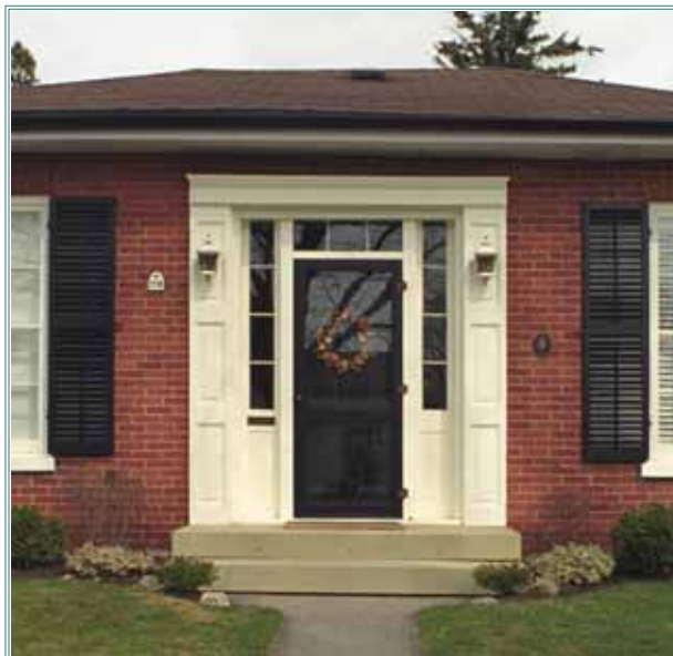
This entrance has been restored and although some of the wood detailing is not authentic, the overall impact is sympathetic with the period of the house.
