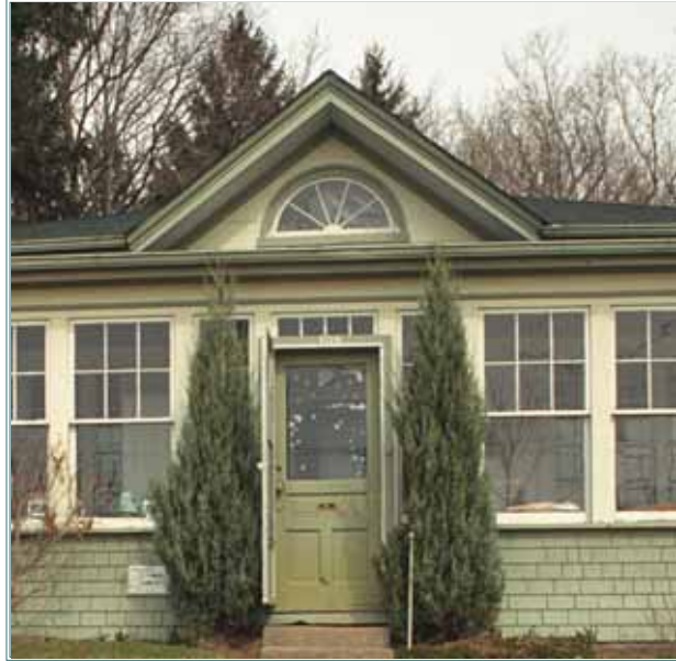
The gable window had lost its divisions but they have been restored. The enclosed sun porch is a much more recent addition and may replace an earlier verandah.
