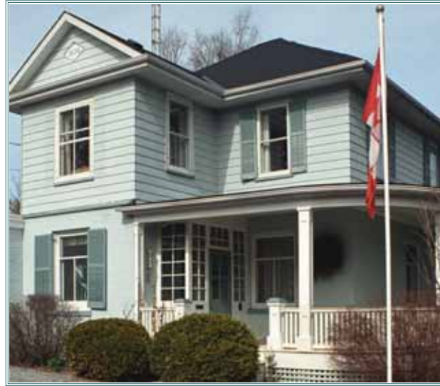
This house was initially constructed as an Ontario Cottage circa 1855. The second storey and wrap around porch were added later in the century.
