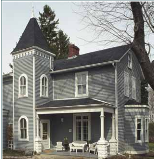
The front two-storey L-shaped section with gable roof facing Yeovil Street was a later addition. Windows have eared architraves which flare out at the sill, a typical detail of 1870's buildings.
