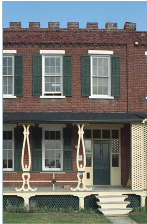
Original details have been restored including original door case and window sash, and fine trellis veranda of lyre design.
