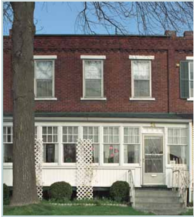
The battlemented parapet has been removed, and the trellis verandah with lyre supports has been replaced with an enclosed porch.
