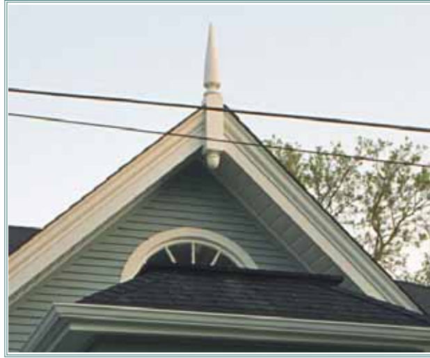
Many of the Ontario Cottages in Port Hope display a finial and drop at the gable peak with a semi-circular fanlight divided into five parts by narrow radiating muntins directly below.
