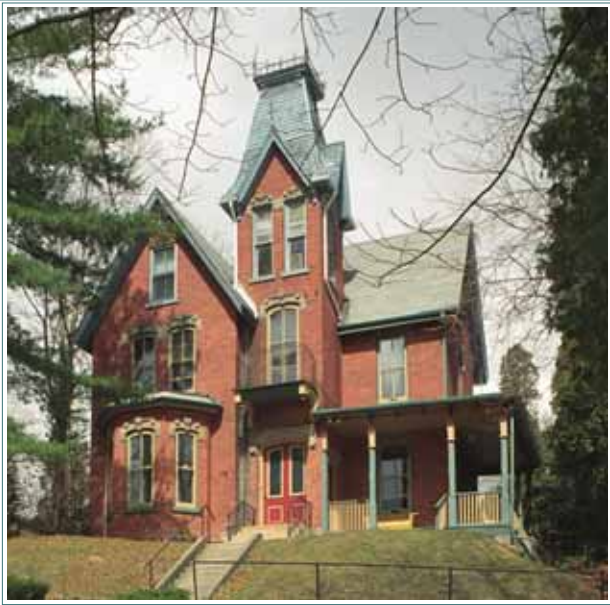
Florid Renaissance detail, multi panelled doors and square towers are typical of the Italianate style. Brown and green were popular colours used on details.
