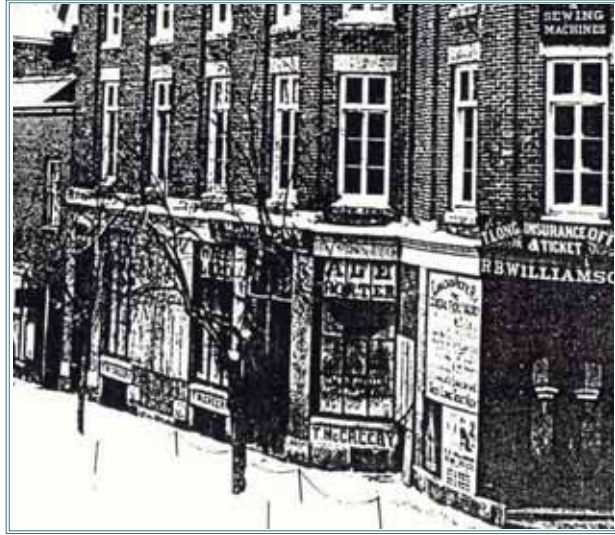
Thomas McCreery sold ale and porter from a shop located in the Robertson Building (35 Walton Street) in the 1880's.
